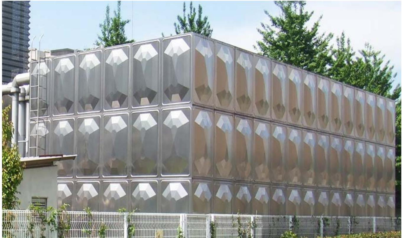
*Modular water tank system made from stiffened stainless steel panels.
