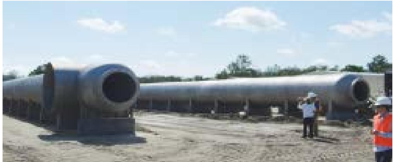
Picture above: Pipework for the hydrogen sulphide removal stage of waterworks.
