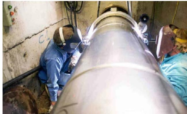
*Stainless steel inserts as a repair solution for underground main supply lines.*
